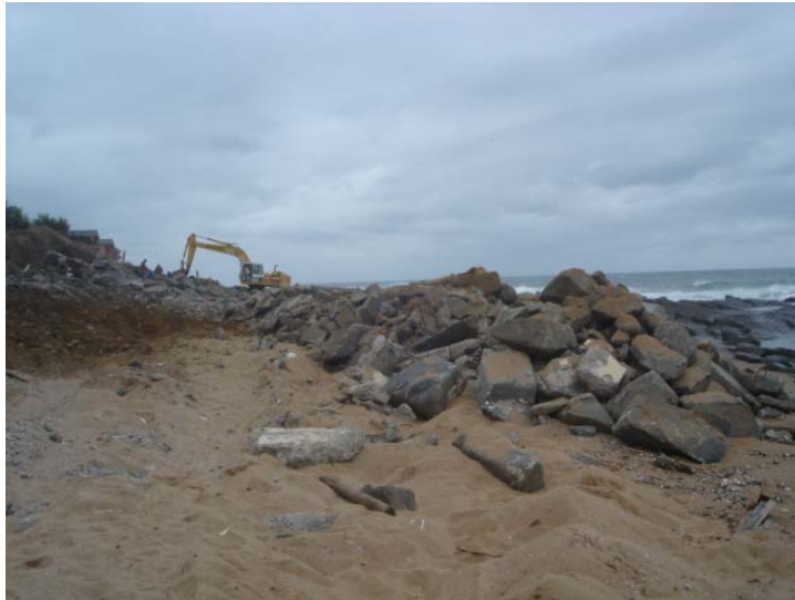
Plate 5 - Suntrap - Local Authority clearing debris for repair of pipe line.JPG
